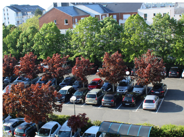
The building's car park located on top of the vertical geothermal probes.
